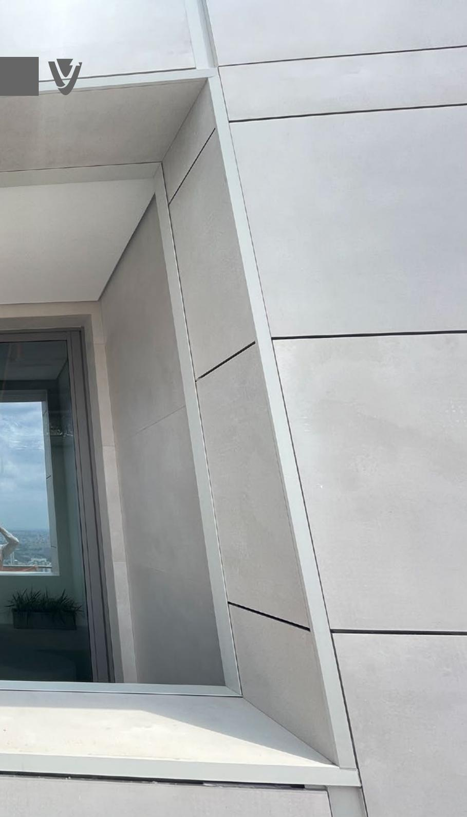
**01** PERFIL BASE FIJADO A LA SUBESTRUCTURA DEL SISTEMA.
